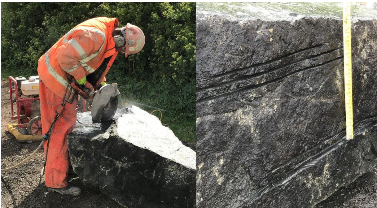
Figure 4: Creation of the distressed features on the granite rock armour.
