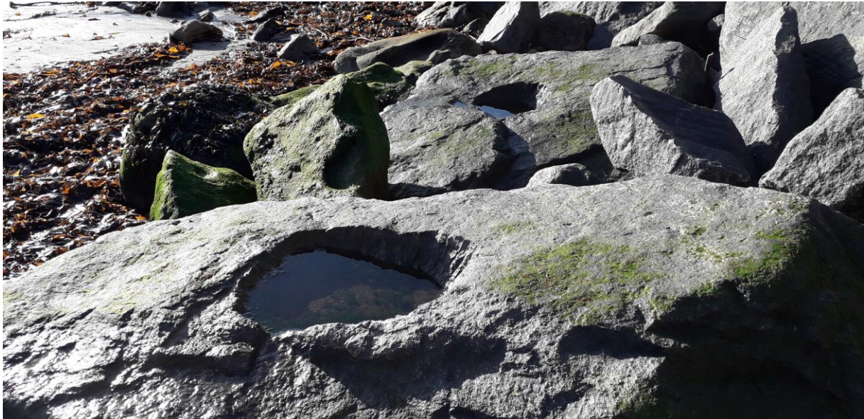
Figure 5: Artificial rock pools cut into the granite rock armour boulders.
